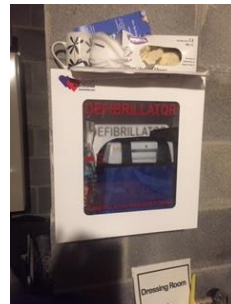
Boiler Room Defibrillator
